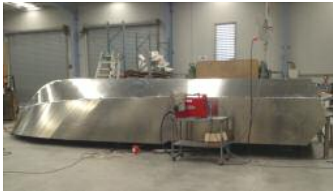
The new vessel under construction.
