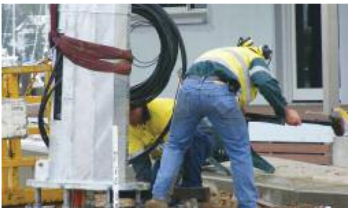
top left: Flagpole being erected.
