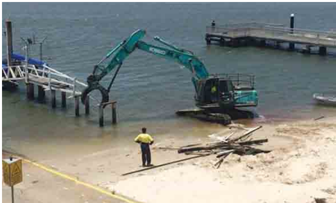
First day of demolition.
