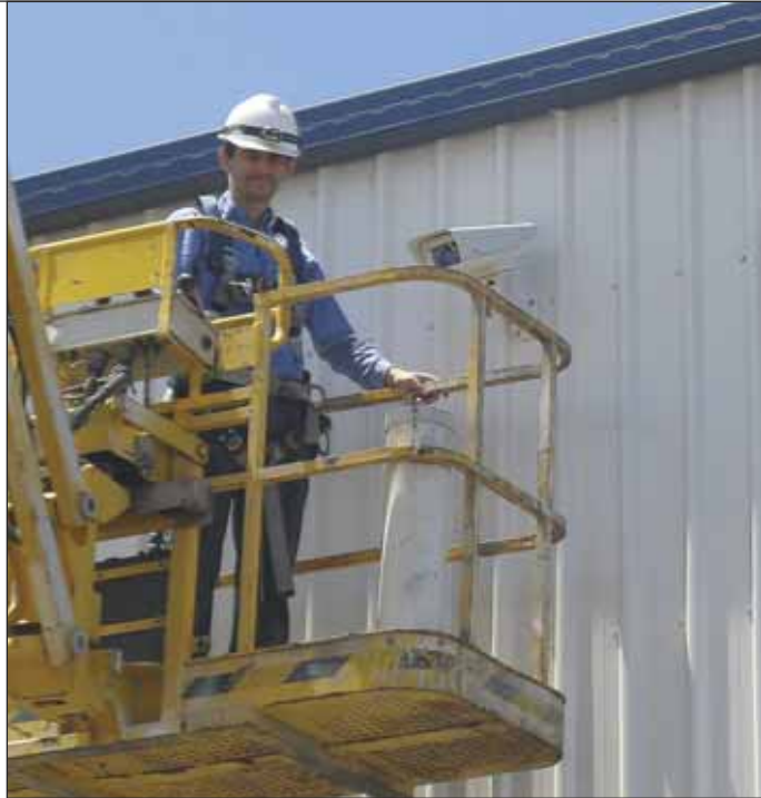
Michael Fleetwood of Jones Communications installing the Axis security cameras.
