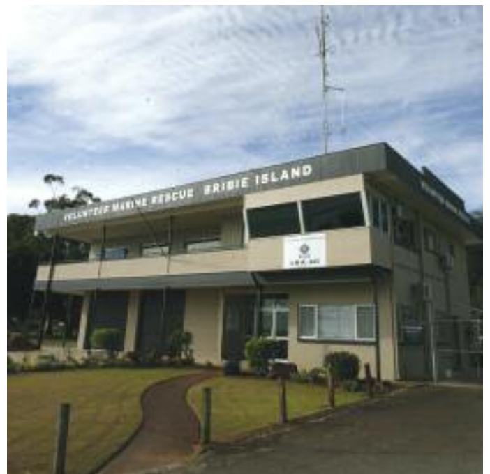
The newly painted Marine Rescue Bribie's Base.
